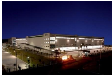
Logistics | Guangzhou, China
