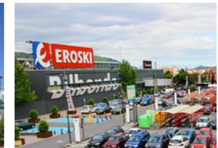
Bilbondo, Handel warehouse, Bilbao
