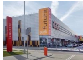
Futura Park, Handel warehouse, Wroclaw
